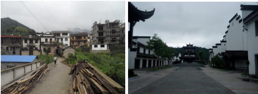
Picture 2 a new house being built in Zhenggang village, Tangkou town
